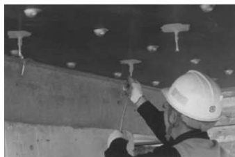
(b) Injection of epoxy
