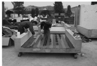
(a) Bonding of FRP sheets
