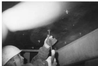
(a) Installation of anchor bolts
