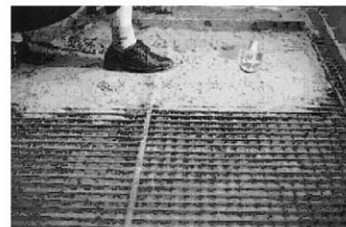
(b) Application of polymer mortar overlay
