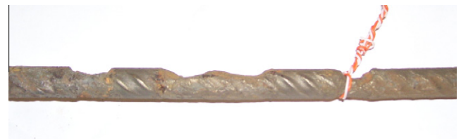
Fig. 4. Appearance of the corroded steel.
