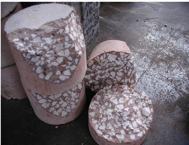
Fig. 16. Fractured concrete by explosive spalling (observed in experimental studies conducted at The Hong Kong Polytechnic University, 2003).
